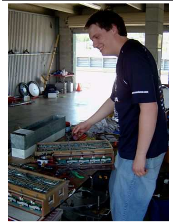
Eli continues work on the battery monitoring system.
